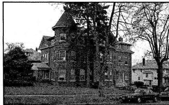
House at 2419 F Street as an example of Queen Anne architecture (DO09:0187-001)
